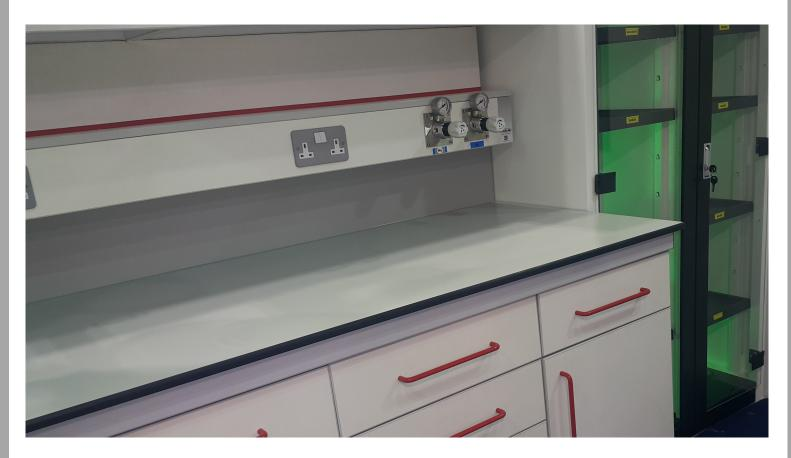
·Laboratory equipment's require clean, particle free environments in order to provide accurate results. Typical gases for these applications include high purity Helium, Argon, Nitrogen, Instrument Air, Carbon Dioxide, Acetylene and Hydrogen. Every component in the line, including the line material needs to be carefully considered for the application to ensure safe use, as well as accuracy and reliability.
